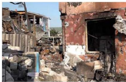
Extensive loss: A damaged private house following a Ukrainian drone strike in Novorossiysk in Russia on Wednesday. REUTERS
